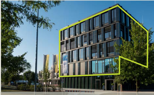
// PV façade at ZSW institute building
